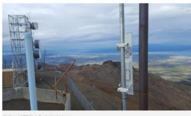
The AARC wrestled with establishment of a high-speed mesh network for several years. The Broadband-Hamnet™ (BBHN) group developed a means to use off-theshelf Linksys WRT54G/GL/GS wireless routers by developing firmware that changes the way the RF decks in these units work. Instead of operating as wireless access points, the radios were used to communicate with other nodes to build an automatically configuring mesh network.
