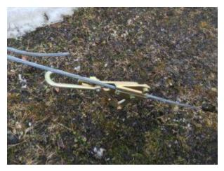
TJ climbed the tower and Dave acted as ground crew. They used the two Klein Tools "Chicago Grips" that TJ purchased from KF7P MetalWerx to get the guy line down. Once they disconnected the bottom end, they laid the guy wire along the vertical face of the tower and TJ went up to about the 40' level and "whipped" the stray wires on the guy fittings so it (hopefully) won't snag the SAMS loop again.
