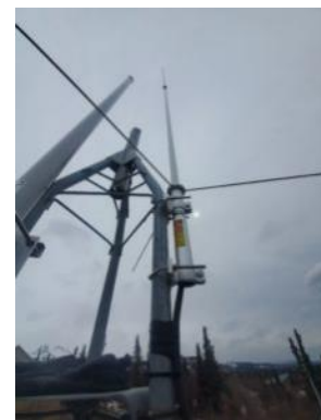
New antenna for 220 MHz Repeater
