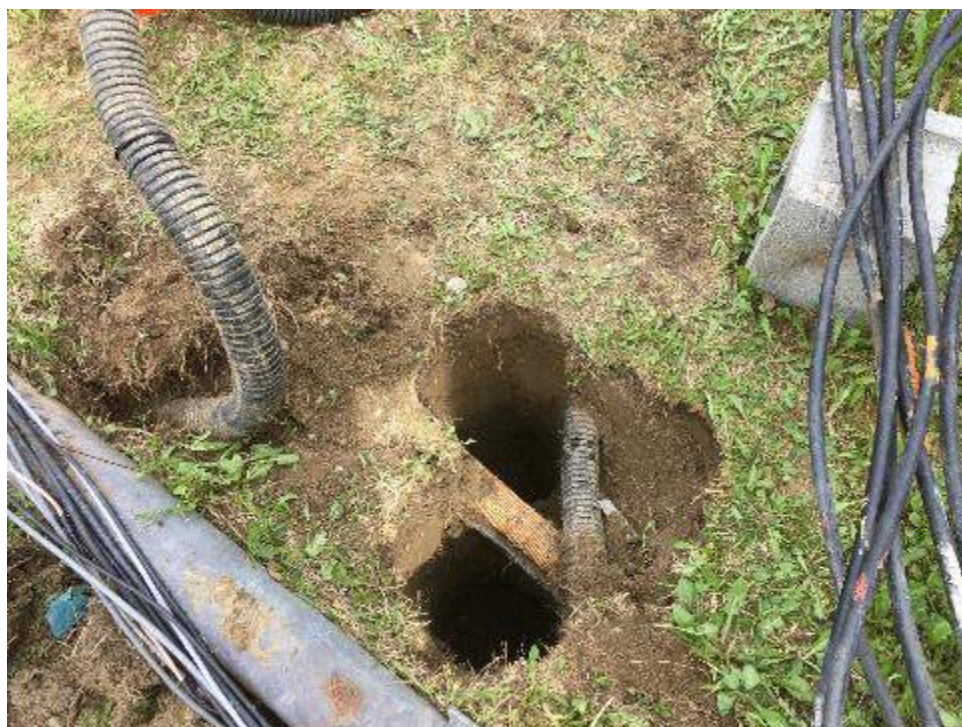
MULTIPLE CABLES AND INNERDUCTS HAVE BEEN IDENTIFIED
