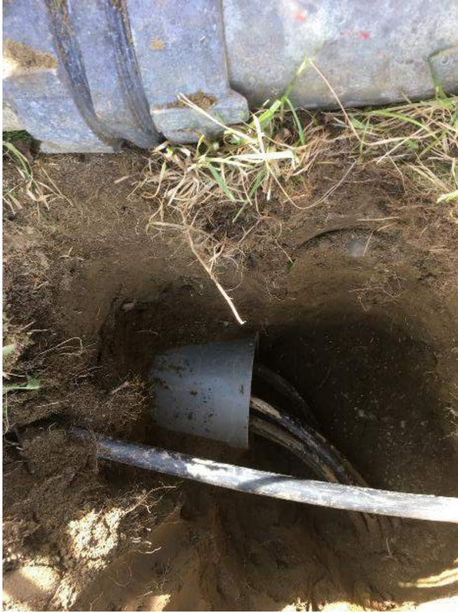
SIX INCH CONDUIT AT 24" BELOW GRADE, WITH 3/C 4AWG DIRECT BURIAL POWER CABLE ABOVE
