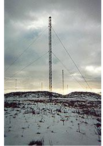
One of the many rusting tower farms on Shemya Island. The sky bears witness to Bering Sea and Pacific Ocean storm fronts moving in.
