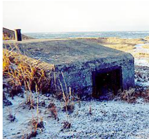
One of dozens of concrete pillboxes, relics of WW II, that litter Shemya Island.
