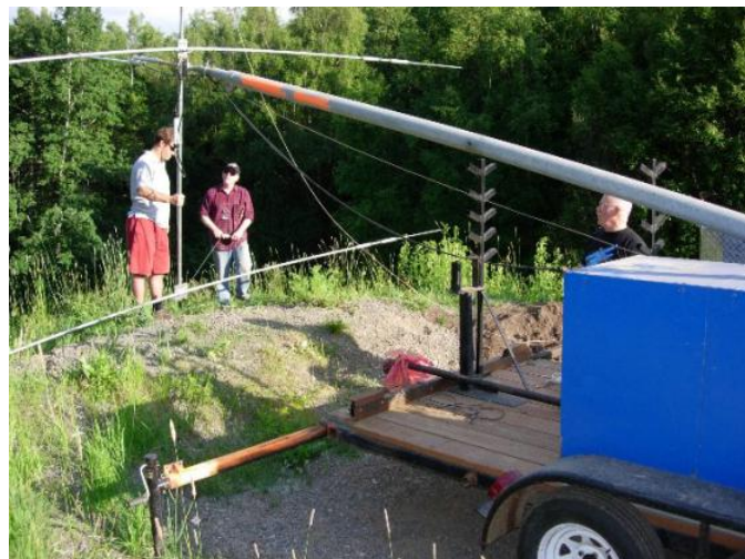
Here the HF beam for the SSB station is about to go up. Luke Smith, KL7LK, TJ Sheffield, KL7TS, and Mike O'Keefe, KL7MD are visible in this picture.
