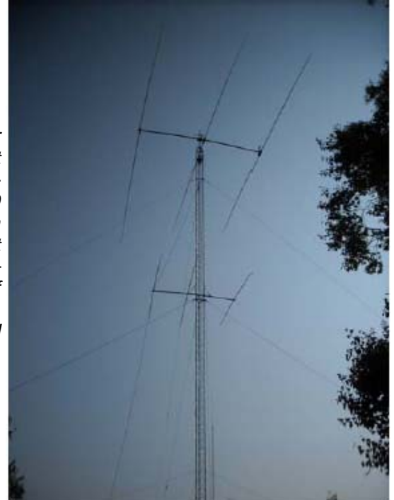
The 40 meter high beam at 180' and a 3-element 20 meter beam fixed on JA at W1AW/KL7 – the station of K L 7 R A . (Photo - Ward Silver NØAX)
